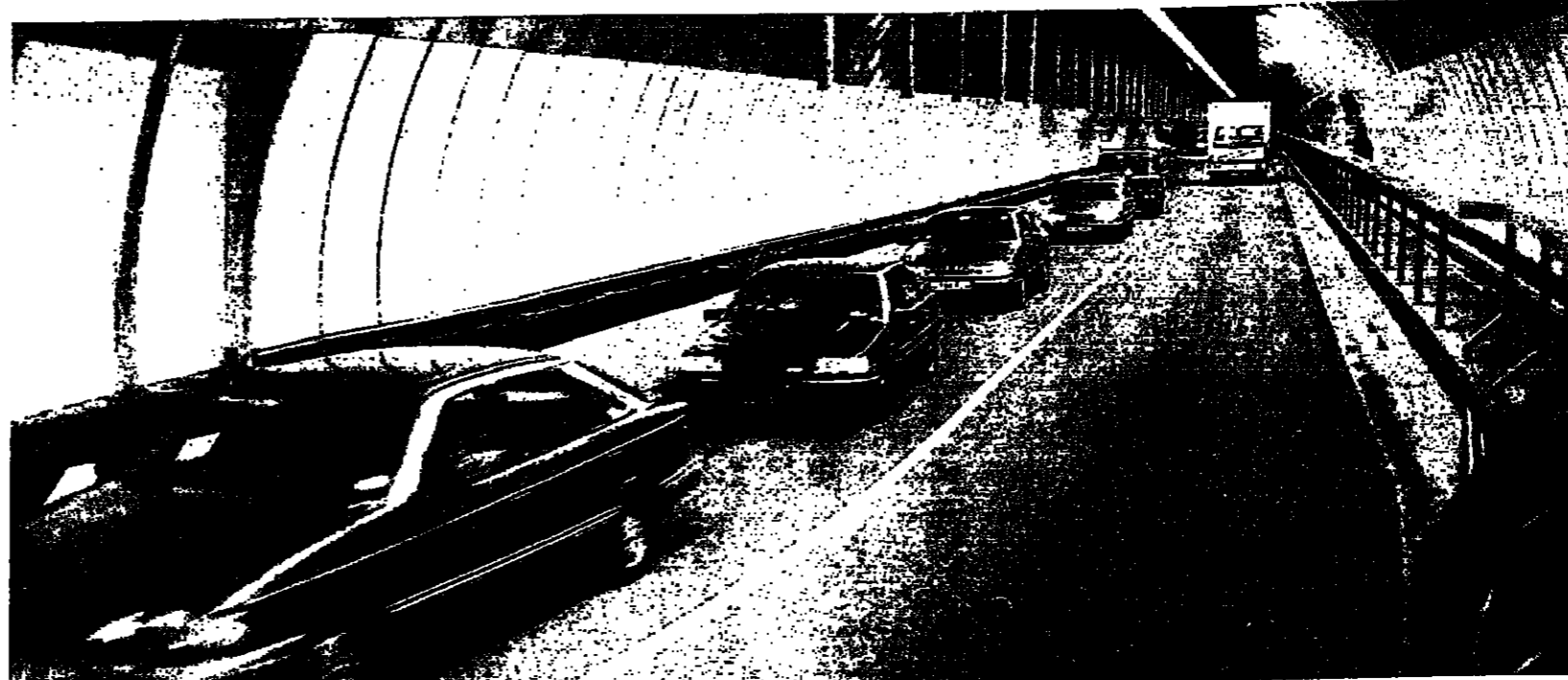
Not always small scale: highways will yield big schemes for local authorities who are responsible for most road, bridge and tunnel maintenance
